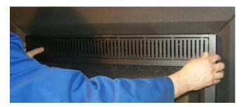
5) Secure bottom of screen using 1 screw on each side into the brackets fixed onto the firebox in step 3.
